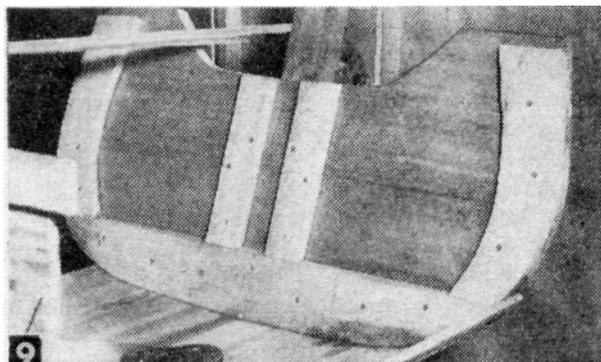
Forward side of transom. Note cheek pieces and strip planks bedded in casein glue around edge.
